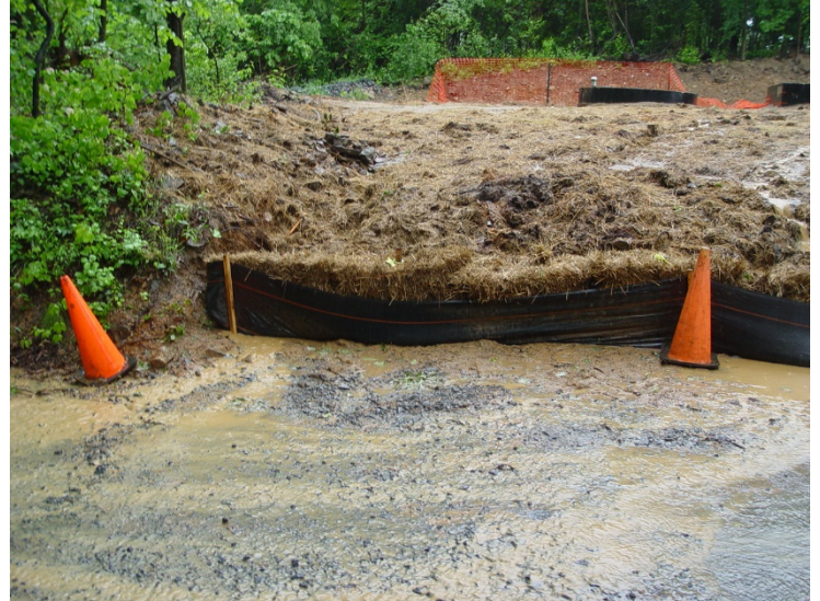
New emphasis on preventing and correcting Erosion & Sedimentation failures at construction sites.
