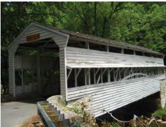
Historic Knox covered bridge in Valley Forge National Historic Park. This landmark is vulnerable to increasing stormwater flows.
