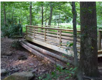
The new bridge, installed at the site.
